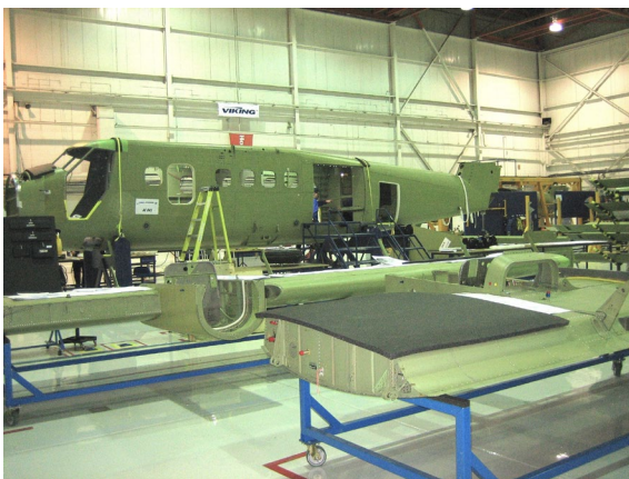
Pictured above: MSN 845 was the first production aircraft through Viking's Twin Otter aircraft assembly facility at the Calgary International Airport.
